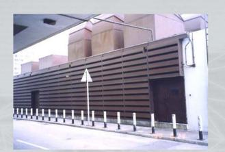
Thickness of acoustic louvres are in 300mm and 600mm in general and could be varied to suit particular application with space and operation limitations. Height and width could be fabricated to suit customer needs, and the general limits for width is 1220mm and height at 3050mm.
